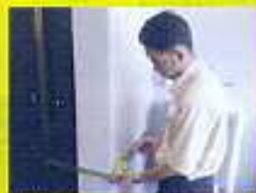
Checking squareness of internal wall
