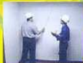
Checking hollowiness of internal wall
