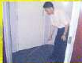
Checking hollowiness of tiled floor
