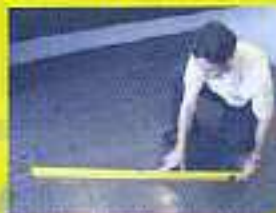
Checking fall of floor in wet areas
