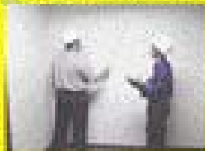
Checking flatness of internal wall
